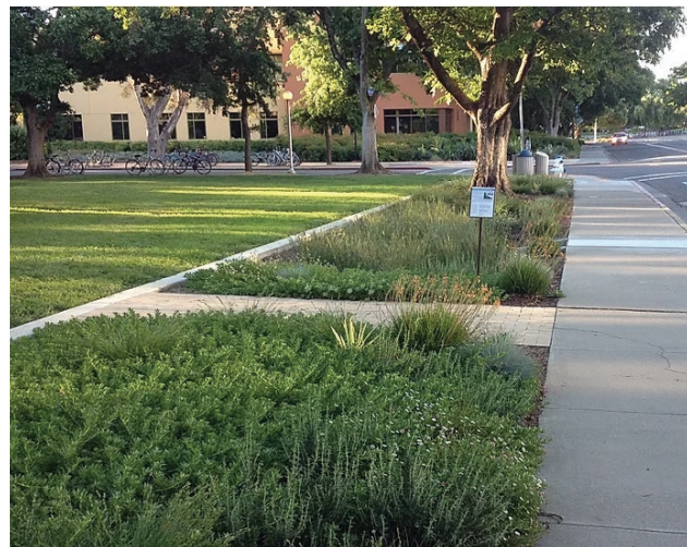
Green Infrastructure Designed and Built by UC Davis Students Captures Stormwater Runoff from the Roadway on California Avenue ( Urban Rain Design )
