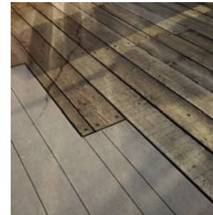
Boardwalk + specialty concrete interface
