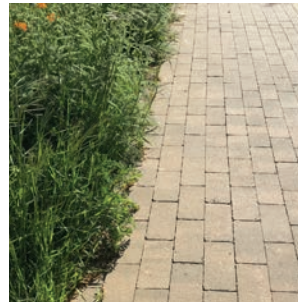
Specialty pavers, such as these interlocking Pavers (UC Davis Arboretum)
