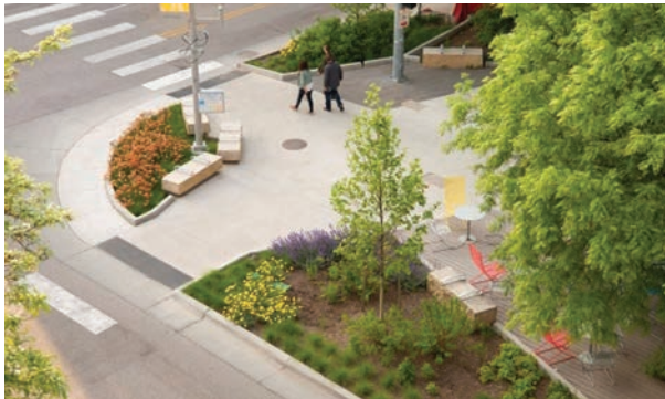
Rain gardens on P St. in Lincoln, NE aid stormwater management, create a road buffer, and include attractive plantings. ( Design Workshop, Inc. )
