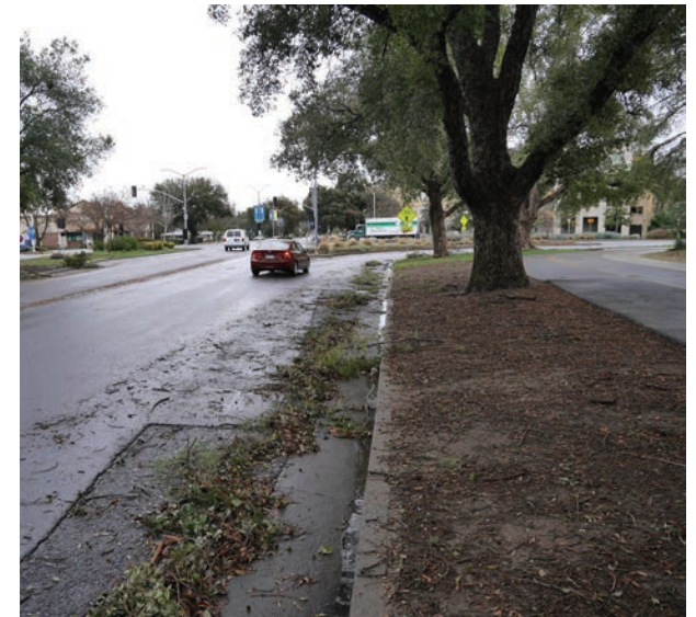
Russell Boulevard Looking East at La Rue
