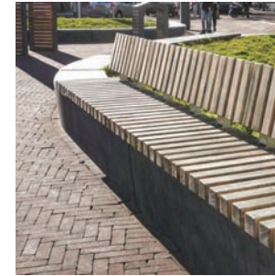
Wood slats + concrete base
