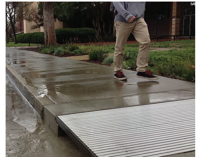
Green Infrastructure Designed and Built by UC Davis Students Captures Stormwater Runoff from the Roadway on California Avenue ( Urban Rain Design )
